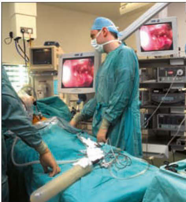
Fig. 1b Overhead boom system in an operating room. Because the equipment hangs from the ceiling, it does not interfere with surgeon and staff movement.
